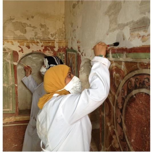
Fig. 6, 7: Graphic documentation before treatment in GB 26 (M9d/SE) assessing the asset and occurring damages. Dry cleaning of surfaces with soft brushes in GB13 (M5/SS).
