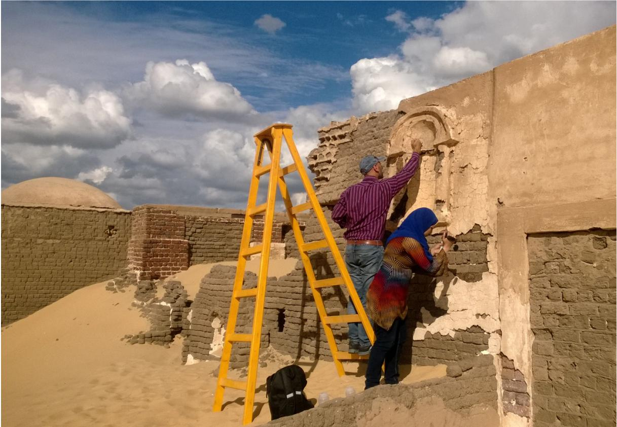
Fig. 10: Pre-consolidation of fragile stucco and plaster edges and the underlying adobe masonry, on the outside wall of tomb house GB 26 (M9d/SE). Photographic documentation during treatment.
