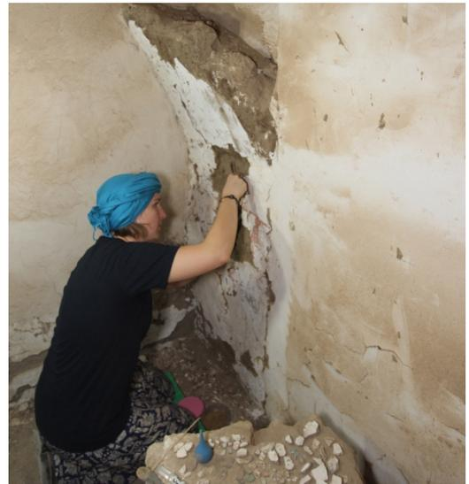
Fig. 8: Conserving the tomb pillar of Hermokrates (GB 20); application of mortar renderings for the painted lime plaster after grouting cavities between plaster and mud brick.
