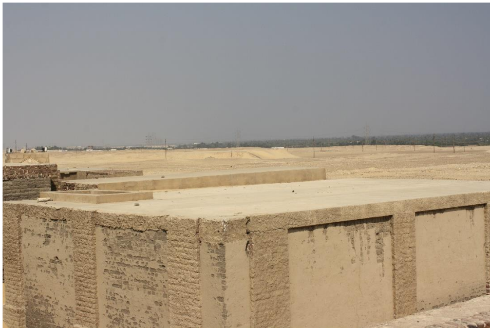
Fig.12: Exterior of GB 11, 12, 13, under one modern roof, supported by added pillars of burnt bricks
