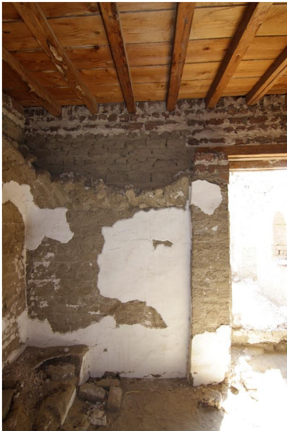
Fig.9: GB 42, wall repaired by adobe and burnt bricks
