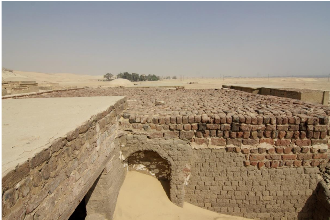
Fig.7: Exteriors of GB 24 (left) and GB 27 (right): walls were completed with burnt bricks, ceilings made of wood and covered by more burnt bricks, or coated with a cement layer
