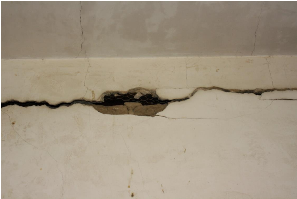
Fig.13: Interior of GB 13, second room, rear wall, a distance was kept between original adobe wall and new roof structure, bridged by metal mesh and plastered with white stiff render
