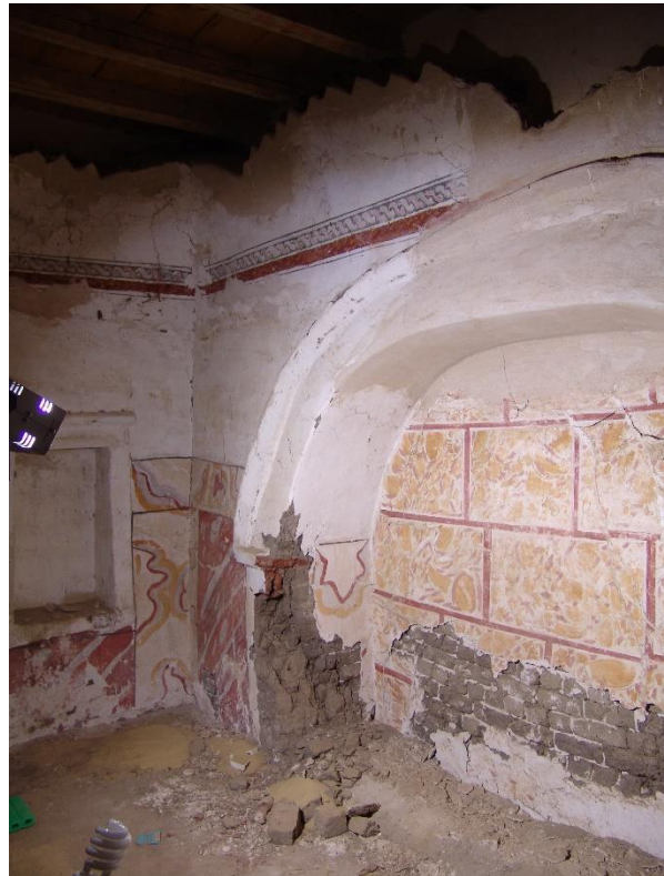
Fig.6: GB27, interior: compressed walls and cracked, detached plaster
