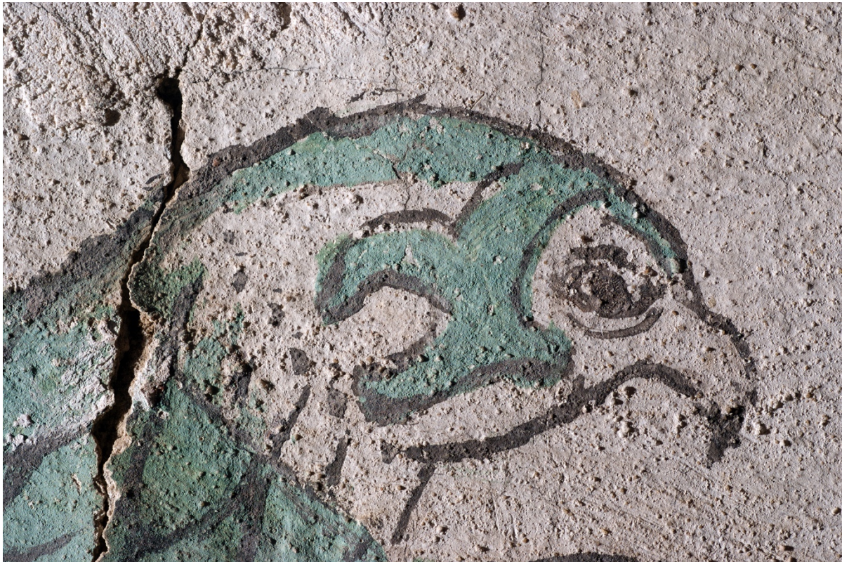
Fig. 6: Detail from east wall of GB33 (M20/SE). The falcon was painted on a thin lime plaster layer. A white wash serves as white background colour. Fine brush stroke impressions in the surface show that the plaster was not evenly smoothed. Like the white wash was applied with a broad coating brush. Width ca. 8 cm.
