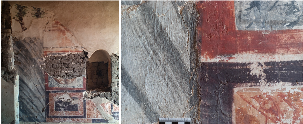
Fig. 10, 11) North wall of GB 26 (M 9d/SE), seventh technological state; plaster stratigraphy differs according to the applied painting technique. The upper- and parts of the lower wall are covered with one lime plaster layer that was white washed and partly painted. The detail (r.) the shows the transition to a two layered plaster stratigraphy in the lower wall zone. The second plaster was only applied in the area of the painted polychrome stone incrustation. The painting being carried out directly on the finely smoothed plaster surface, apparently intended as fresco technique.
