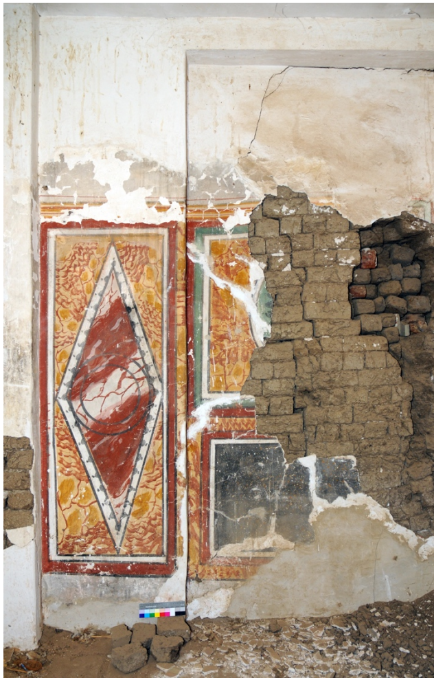
Fig. 12: North wall in GB 13 (M 5/SS), fifth technological stage; two layered plaster in lower wall zone with polychrome stone incrustation wall painting directly on
