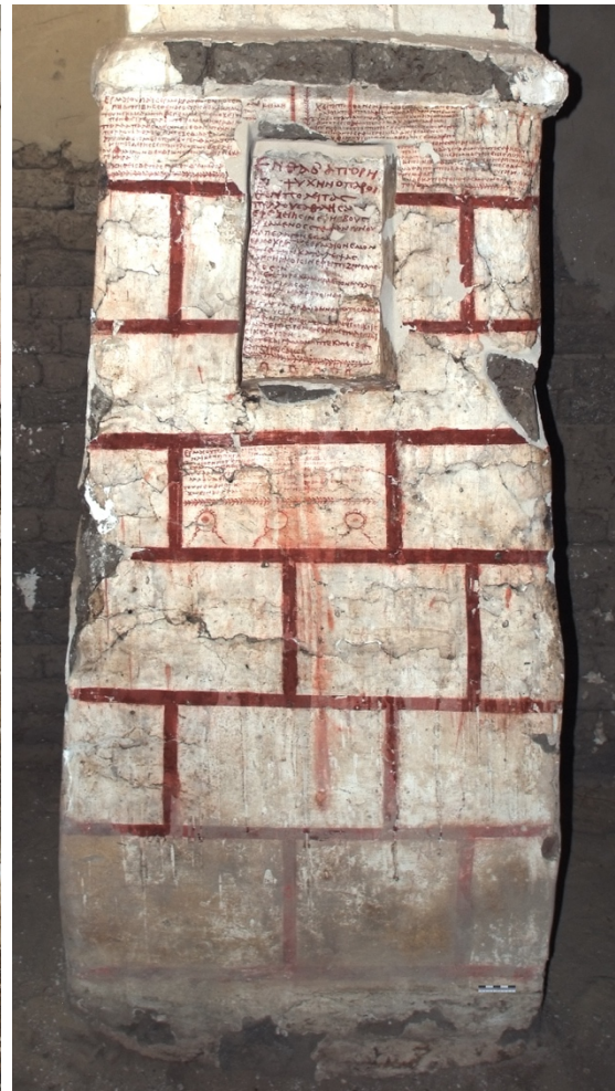
Fig. 13: Tomb pillar of Hermokrates, GB20, lower part of western side, 9 th technological stage; one, in parts two-layered lime plaster on mudbrick
