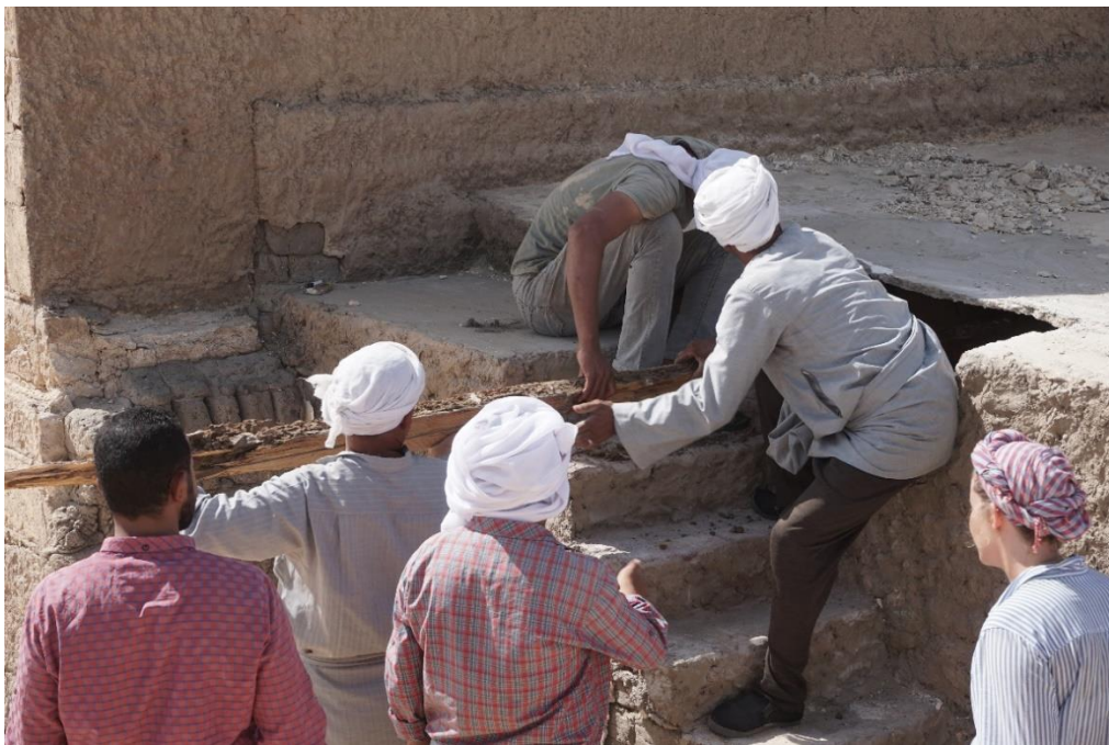
Receiving the rotten beam
