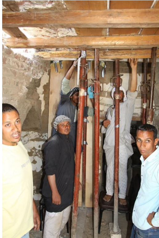
Sliding out the rotten beam
