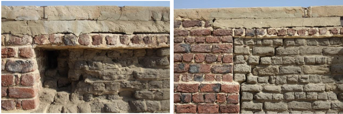
South façade, closing of a hole to prevent animals from settling in
