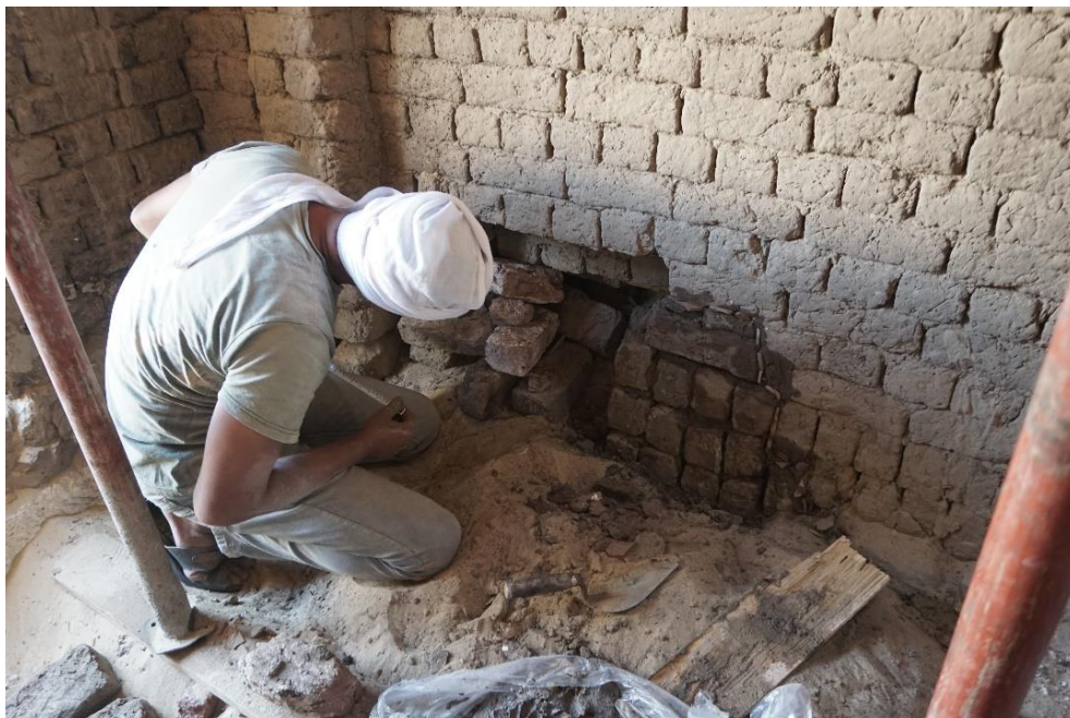
Antechamber, mason repairing the mud brick wall
