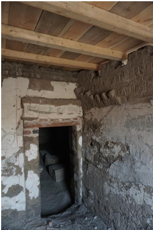
New woodwork of the roof; interior wall relieved of pressure from the roof
