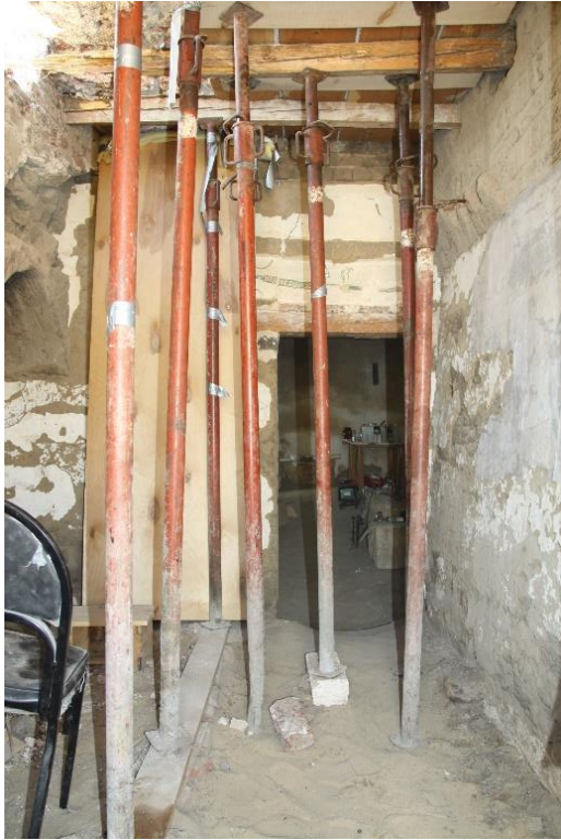
Roof supported by jacks
