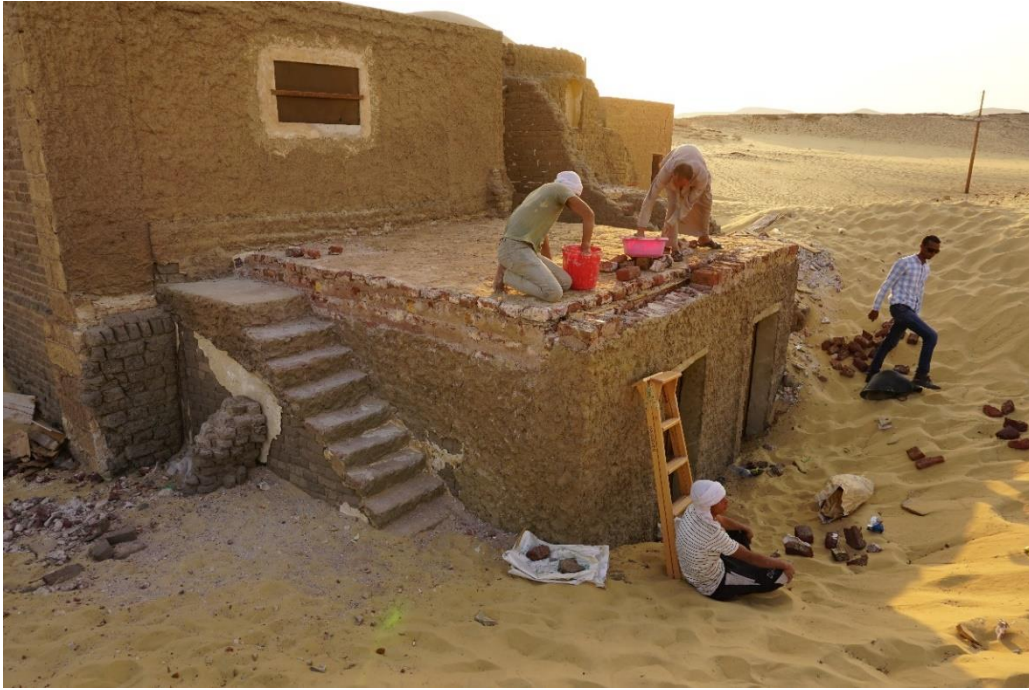
Final work on the new roof: laying red bricks in lime mortar
