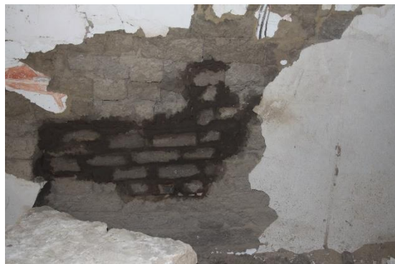
Deteriorated wall in the main chamber, east wall, before and after repair
