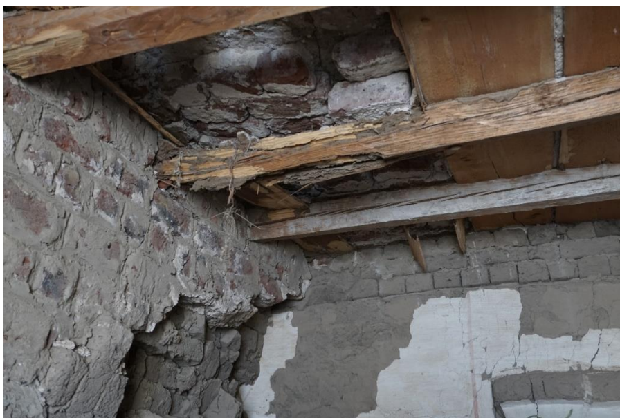
Deteriorated ceiling in the antechamber
