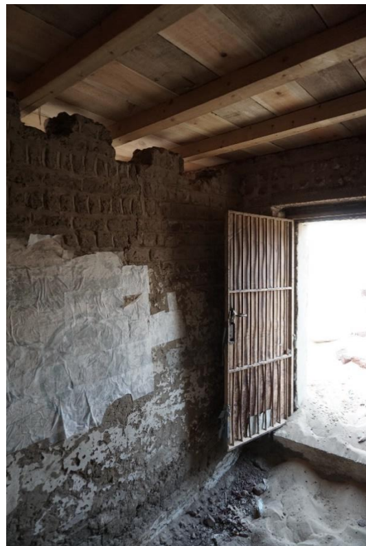
New woodwork of the roof; interior wall relieved of pressure from the roof
