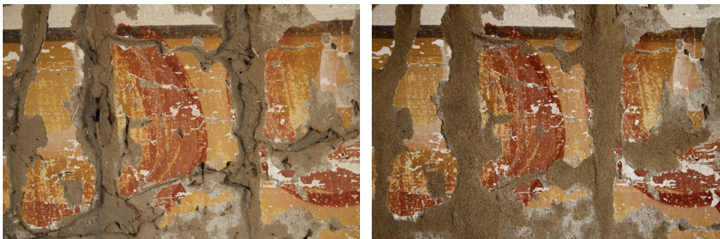
Figs. 09,10: GB24 inside,north wall, before and after application of conservation plaster
