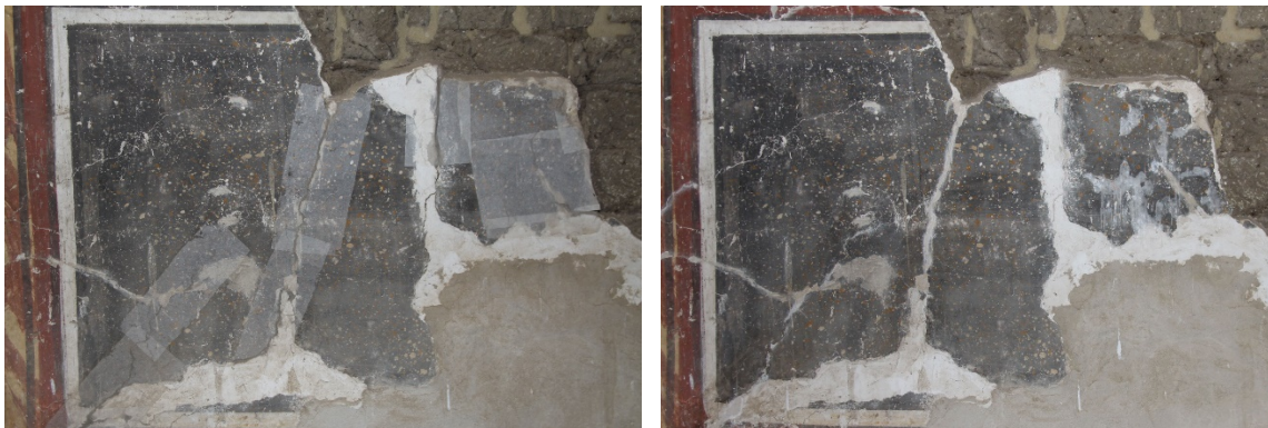
Figs.17,18: GB 13 first room, south-east wall, before and after grout injections; the Japanese paper facing could be removed after stabilization
