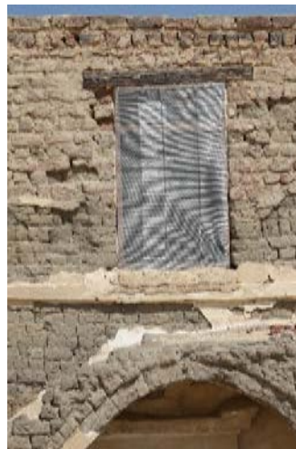
Figs.21, 22: GB 20 west side (Hermokrates) and GB 04 south side, windows were closed with mesh
