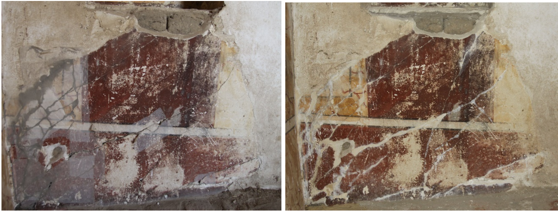
Figs.15,16: GB 16 first room, south wall, before and after grout injections; the Japanese paper facing could be removed after stabilization
